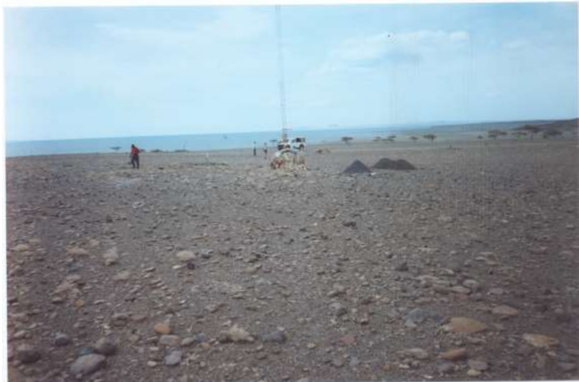
Plate 6: Lake Turkana Windpower mast at Loyangalani.
