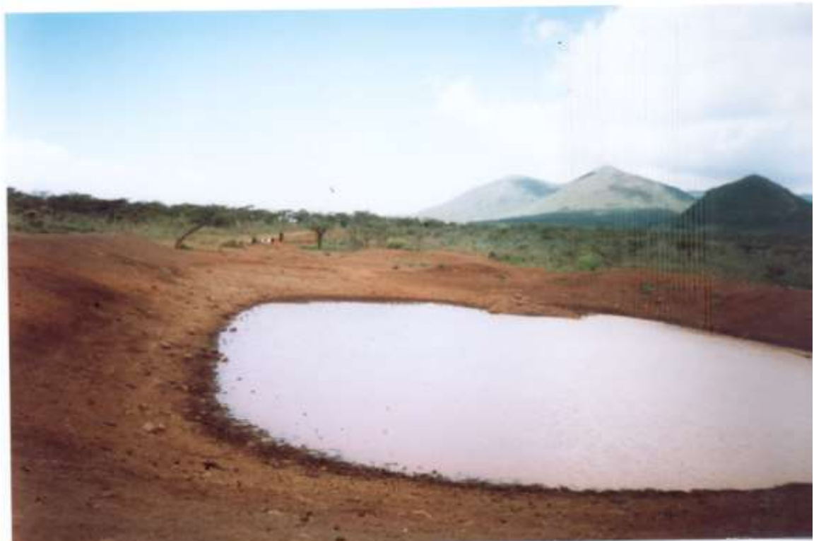
Plate 16: Earth dam for the watering of cattle at the periphery of the project area on the way to Qatab, Mt Kulal region
